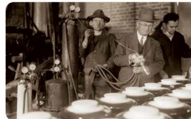
*Metaltzowanie izolatorów W60 / Metal plating of W60 insulators (arch. Photofactory®)*
