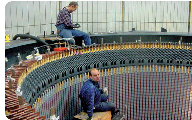
Remont generatora w Elektrowni Porąbka-Żar / Overhaul of generator in Porąbka-Żar hydroelectric power plant
