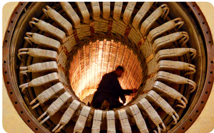
Remont generatora, 1988 r. / Generator's overhaul, 1988
