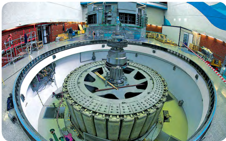
Hydrogenerator El. Czorsztyn-Niedzica w trakcie remontu / Hydrogenerator of Czorsztyn-Niedzica Power Plant during overhaul
