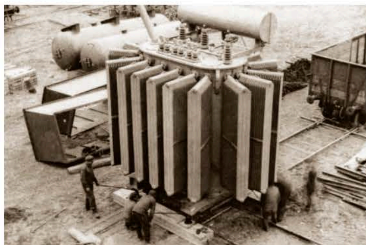
Transport transformatora – 1 maja 1939 r. / Transformer in transport – 1 May 1939
