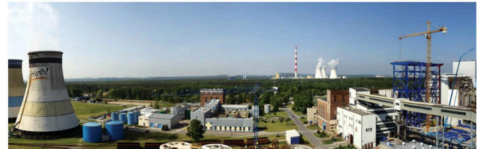
TAURON do końca 2020 r. planuje uruchomić moce oparte na spalaniu biomasy na poziomie 240 MW – budowa kotła biomasowego w jaworznińskiej elektrowni – maj 2011 r. / TAURON plans to launch energy generation based on biomass combustion at the level of 240 MW by the end of 2020 – construction of a biomass boiler in Jaworzno Power Plant – May 2011
