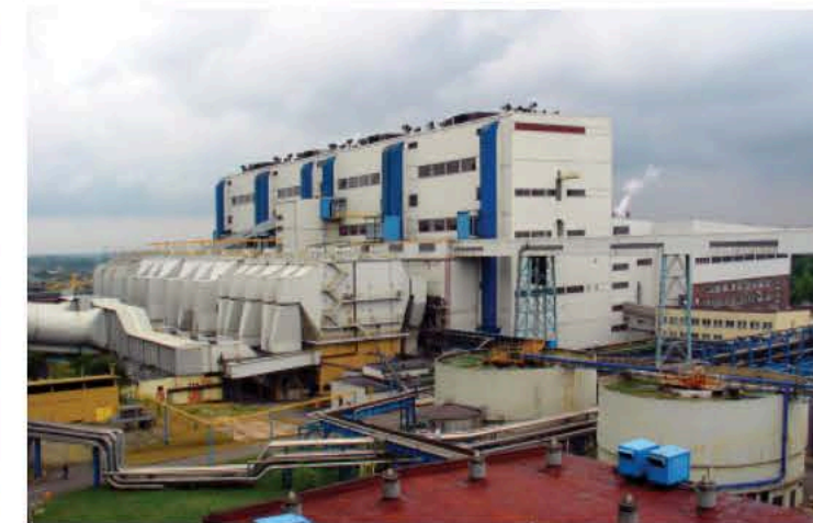
Widok na bloki 225/230 MW / View of 225/230 MW units
